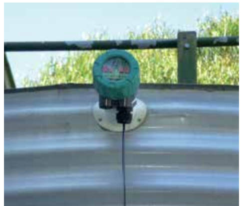
High level switch in plastic pellet silo
